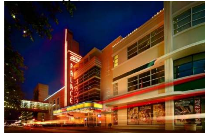
Figure 14.19 Marquee signs should be utilized for theaters and other similar entertainment venues
