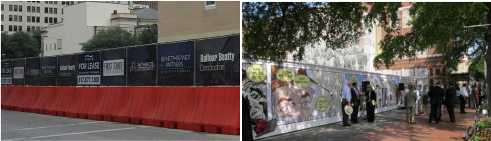
Fig 10-7: Illustrations of acceptable construction site screening.
