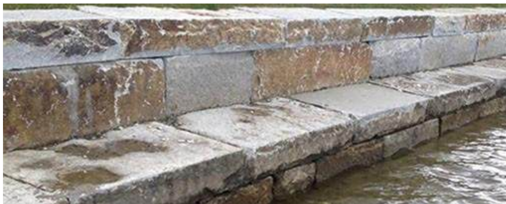
Rough Stone Block Wall/Coping
